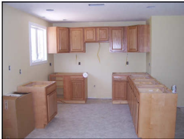
A new kitchen...almost ready!
